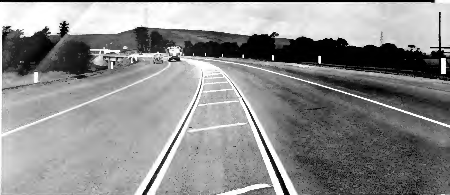
View of stretch of new divided highway on U. S. 101 at Sargent in Santa Clara County
